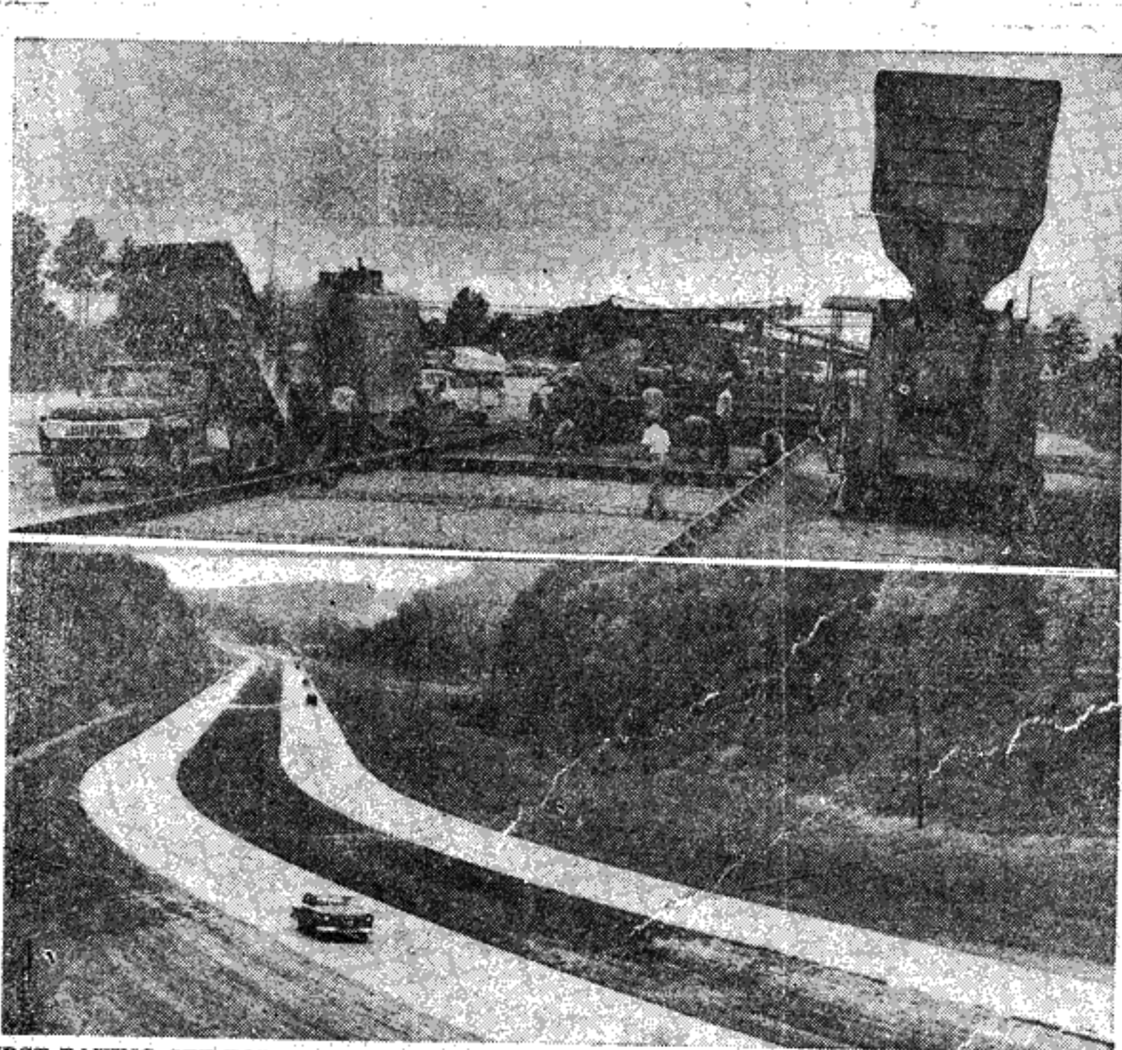
FIRST PAVING SET FOR ALABAMA'S NEW FEDERAL INTERSTATE SYSTEM—Above photo shows 10-inch, heavy-duty concrete being placed on completely new highway location, 20 miles north of Birmingham, near Warrior—first actual paving in Alabama's new super-highway program. Lower photo shows how new highway will look upon completion. This four-lane section on U.S. 31, north of Birmingham, was completed last year and Director Herman Nelson has announced it will be incorporated into new Federal Interstate System. Alabama has over 900 miles on Interstate System. "Limited Access" requirements will be added to above highway at later date.
